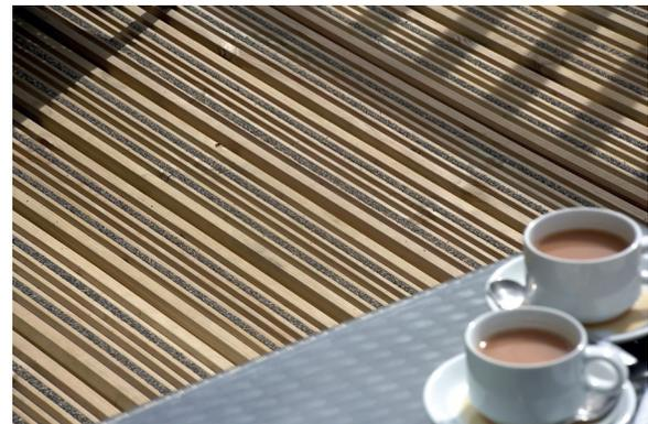
The process transforms timber deck boards into fully tested and safe non slip surfaces. The specially formulated combination of resin and aggregate has been designed to work on all specifications of timber decking and is a robust solution to the hazards posed in slippery conditions.
